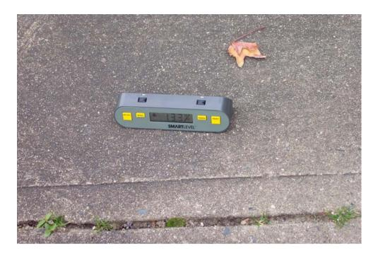
b. There are transistions from the street to the curb cut of 1 inch contrary to ANSI section 403.4 and ADAAG section 4.3.8.
