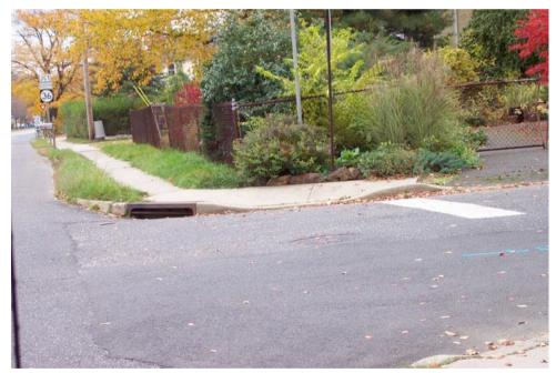
c. The sidewalk adjacent to the curb cuts have more than 2% slope and will make a wheelchair travel in the direction of the slope contrary to ANSI section 403.3 and ADAAG section 4.3.7.
