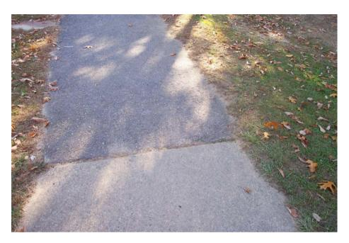
8. At the end of the sidewalk there is no curb cut, contrary to ANSI section 303.4 and ADAAG section 4.7.1.
