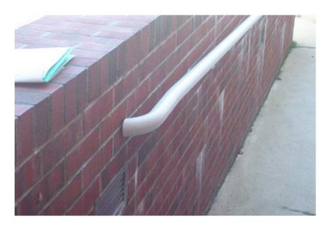
f. The slope of the first section of the ramp to the landing is 9.8%, contrary to ANSI section 405.2 and ADAAG section 4.8.2.
