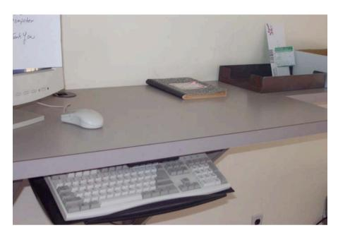
c. The side counter next to the computer measures 45 inches above the finished floor, contrary to ANSI section 902.3 8 and ADAAG section 4.32.4.
