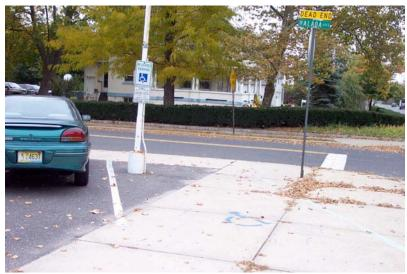
2. The front entrance ramp has a slope of 6.3%, contrary to ANSI section 404.2.4.5 and ADAAG section 4.16.6.
